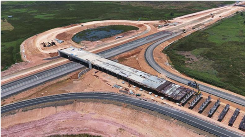
Gambar 18 Area Interchange Jalan Tol
