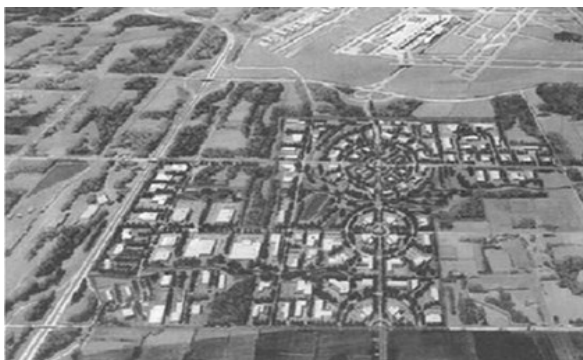
Gambar 6. Detroit Metro Airport (DTW) di Michigan, AS
